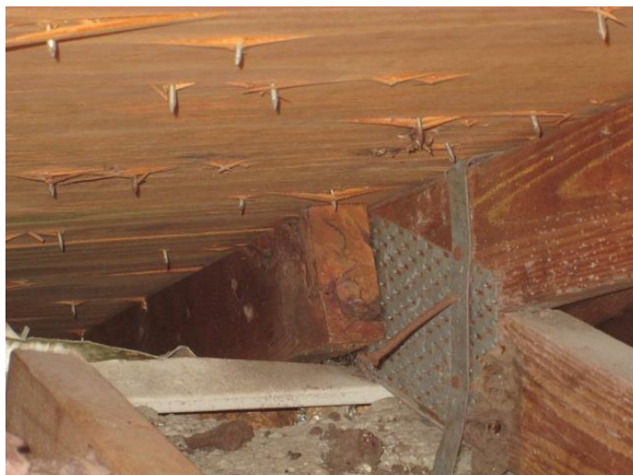
Roof to Wall Attachment
