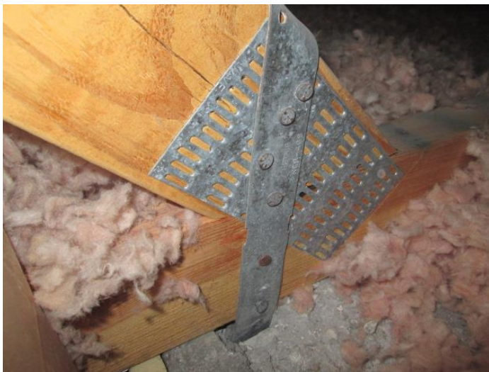
Roof to Wall Attachment
